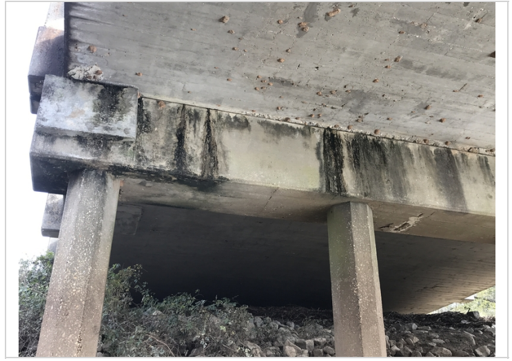
Cap - Bent 5 back: Patched/rebar exposed
