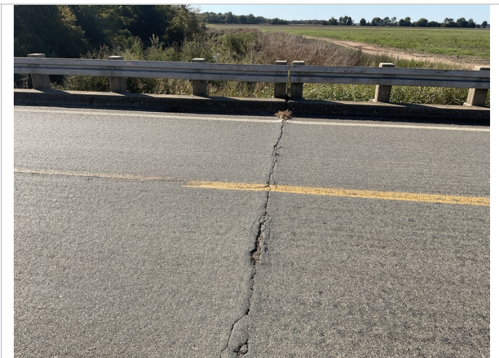
Bent 2 joint seal has debris impactation due to asphalt overlay. Common on all joint seals.
