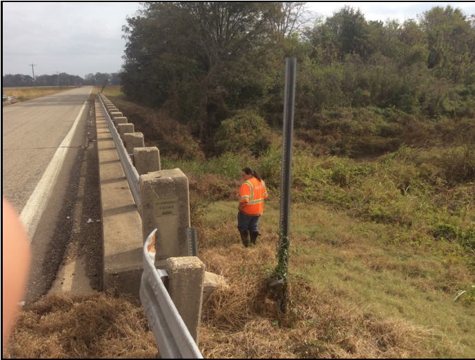
Object marker and logged mile signs missing on both ends of bridge
