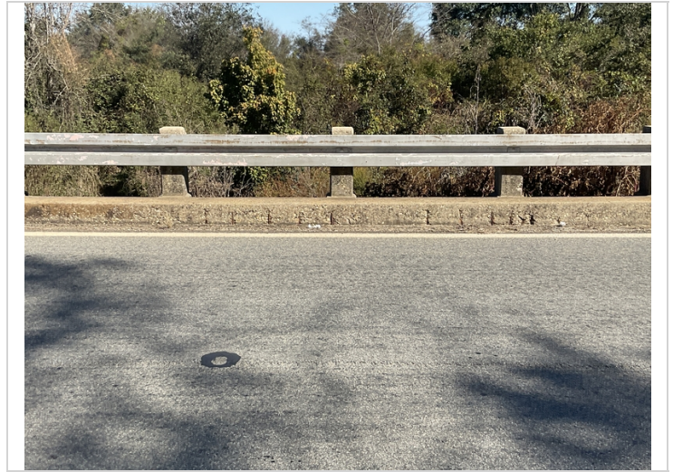
Span 5 right concrete curb has exposed rebar.
