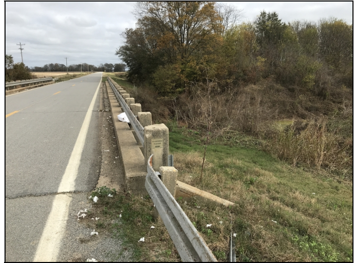
Log mile sign - Bent 1 right: Sign missing
