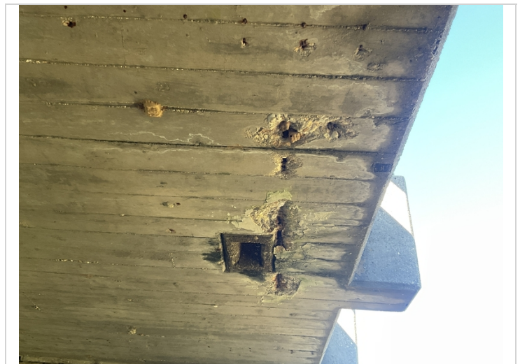
Bent 2 left soffit at drain opening has minor spalling with exposed rebar.
